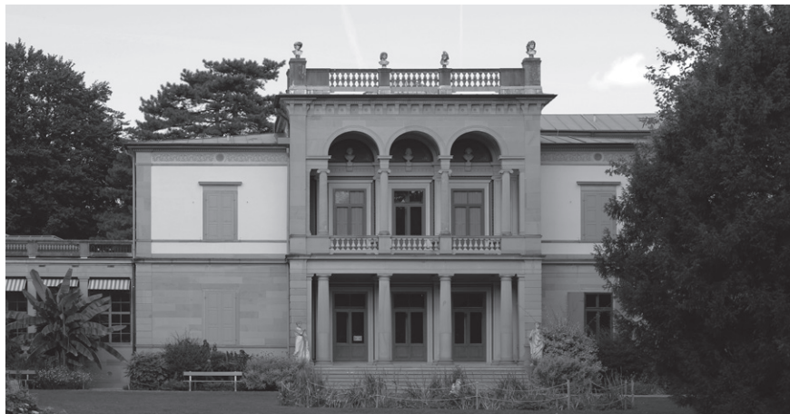
Museum Rietberg, South Facade, 2023
