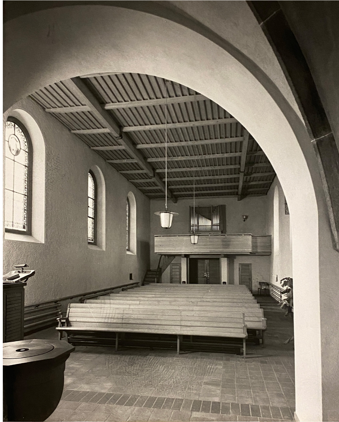
Interior of the Old Church after the renovation by Werner Moser, 1942.
