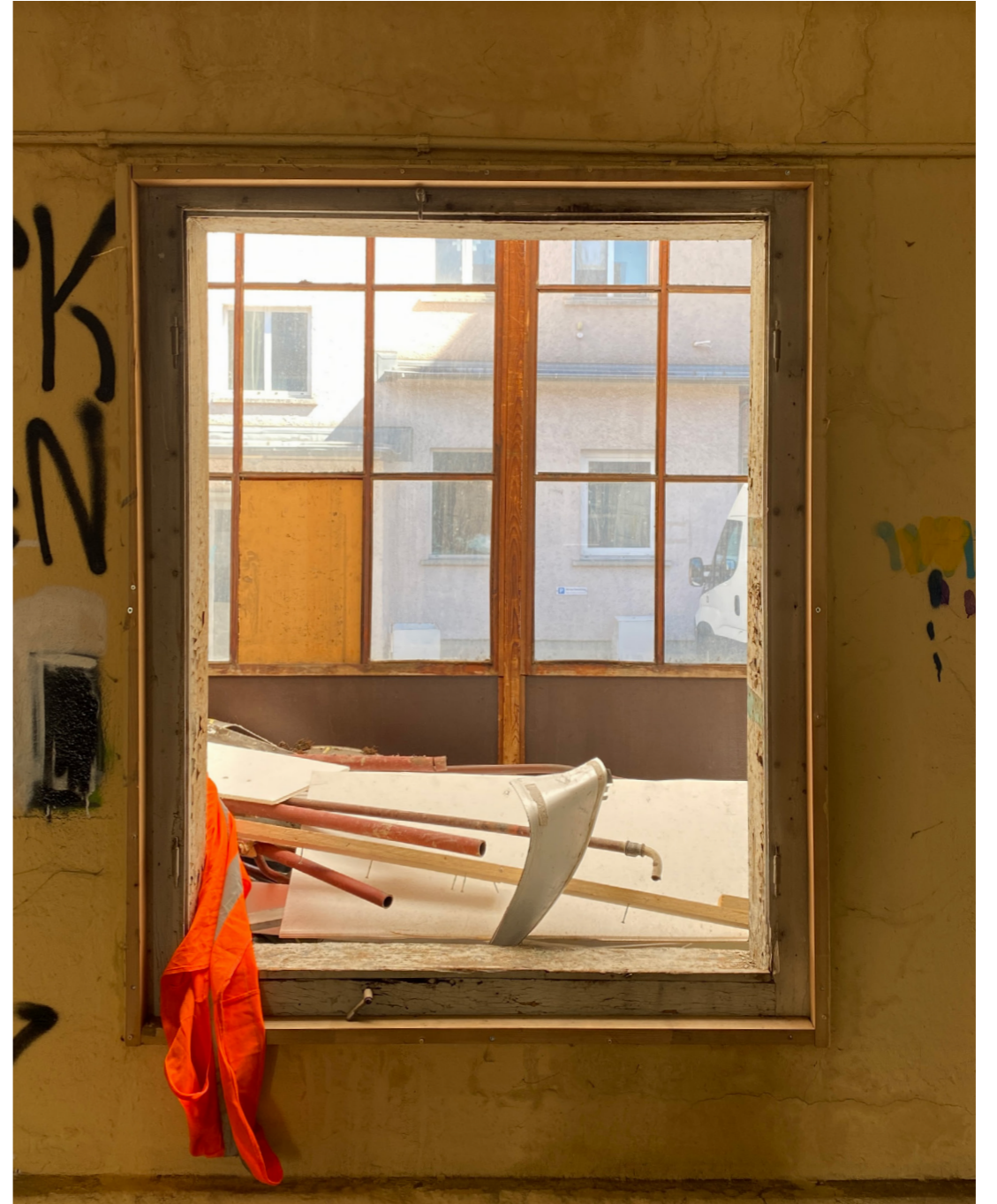
Abandoned building at Lindenplatz, Badenerstrasse 686.
