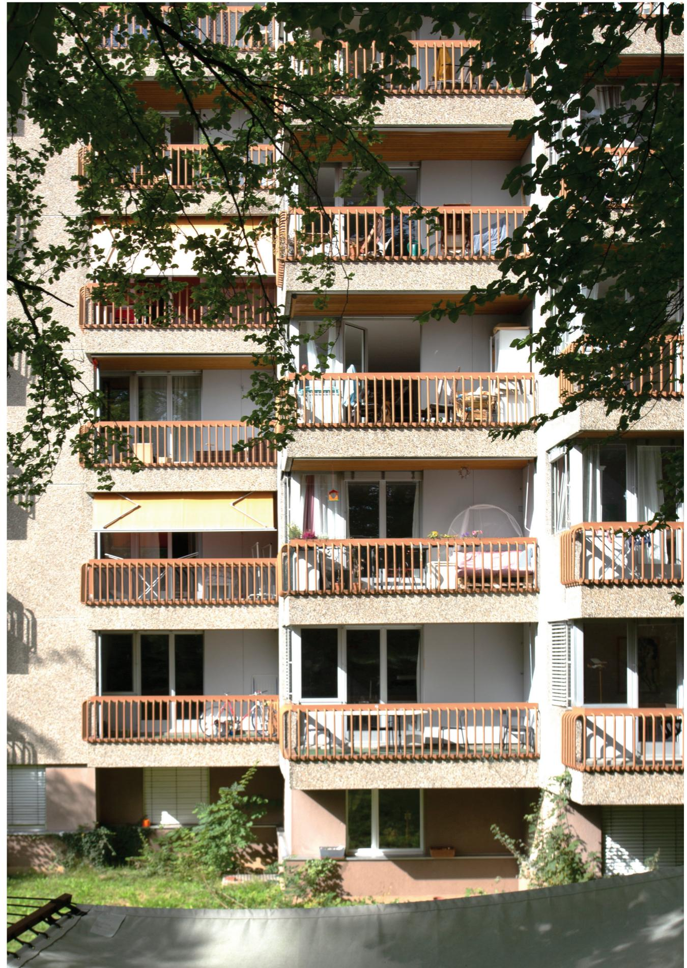
The rectangular shapes seem to be stuck to the façade. The orange-brown-ish metal rail wraps around it and is fixed to the concrete slab. The corner detail is quite distinguishable.
