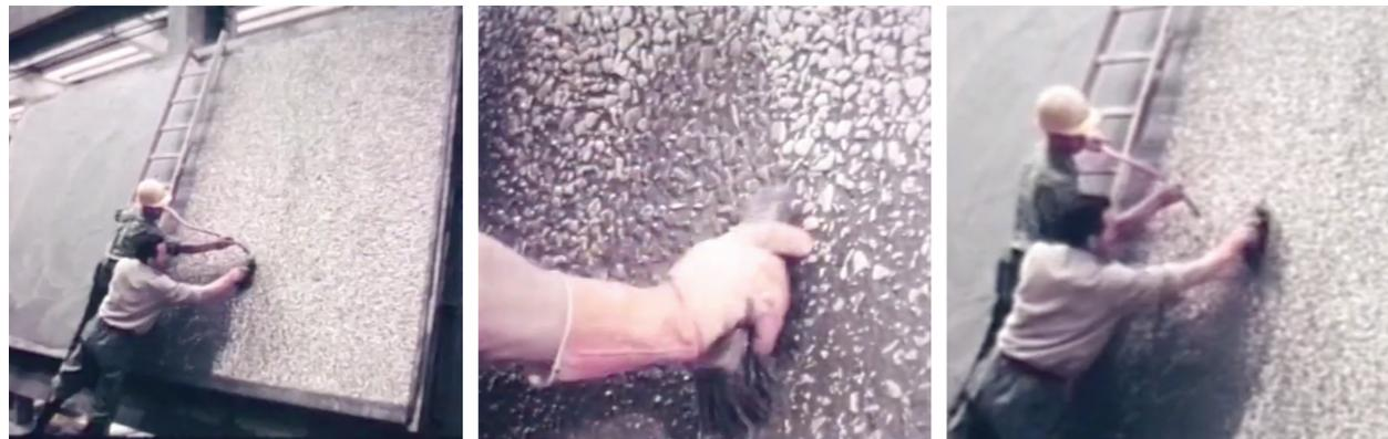
1 Shortly before the top cement skin is hardened, it is washed off with a weakly flowing waterjet.
