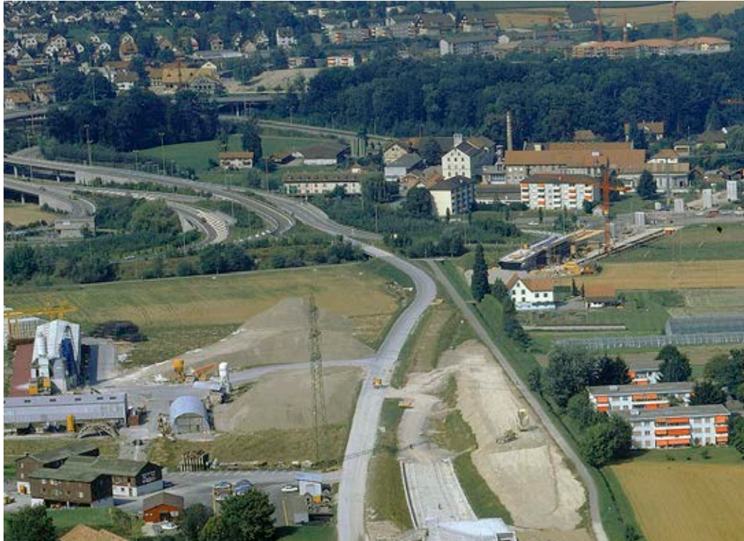
unkown, 1985 Excavation piling up (left) Gärtnerei Kohler (right)
