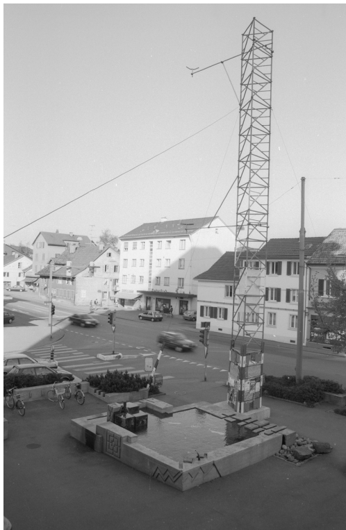
View on the ‚Marktplatz‘ with the sculptural fountain and a scaffolding next to it. March 1990
