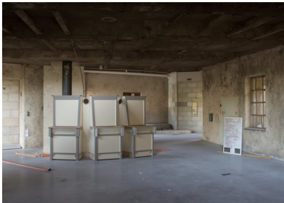
concrete construction, construction site
