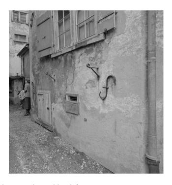
On old manor houses, the treble clef flashes at the corners of the buildings. It pulls and holds the façades together, keeping them in subtle tension. It transforms necessity into a mark of distinction. Together with its relatives scattered throughout the village, it creates a network that blends function and design.
