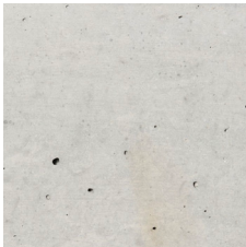
Beton Structures, Extension
