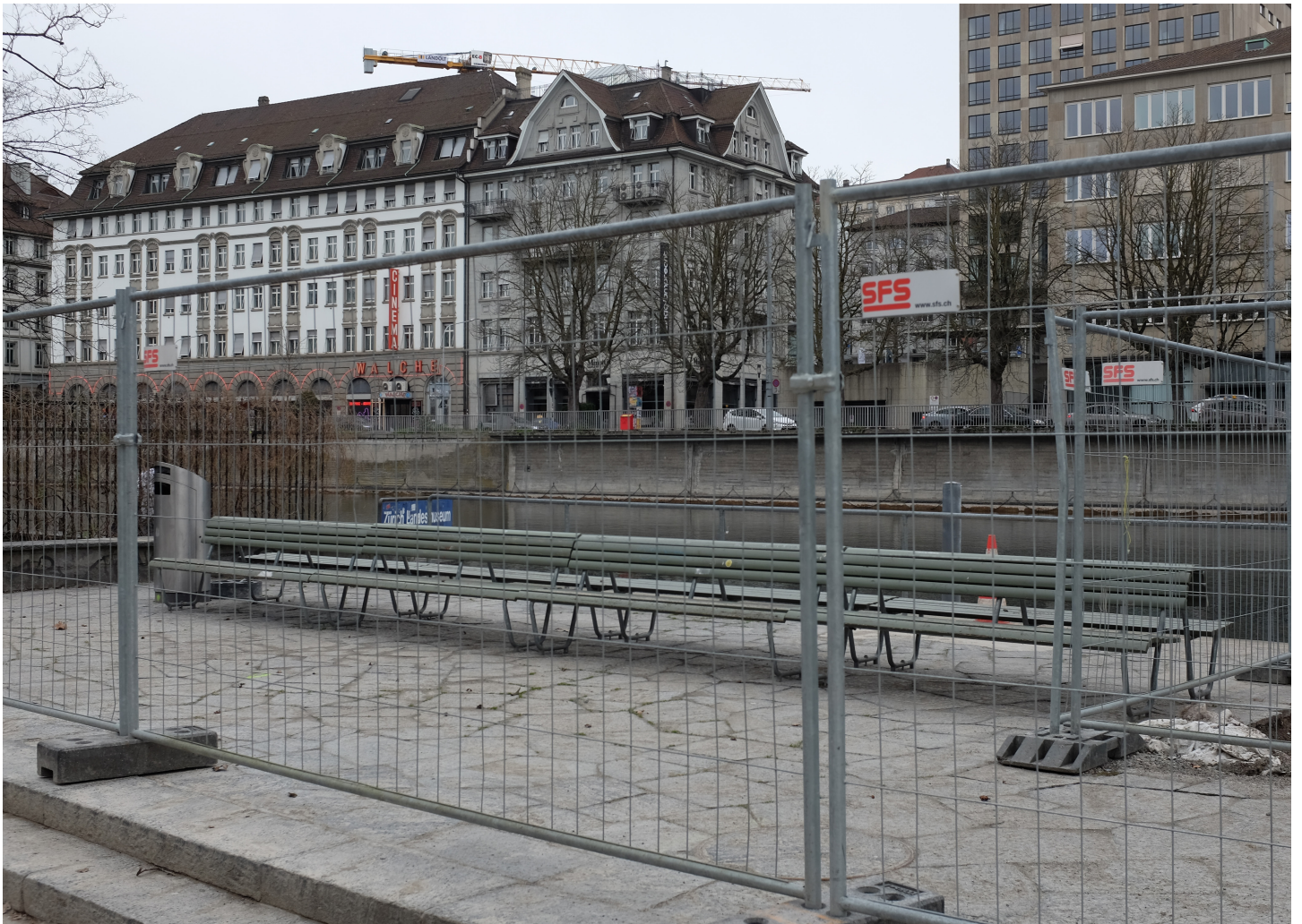
Fig.1.16: A set of public benches fenced in due to a construction site next to it making the benches unaccessible for anyone.
