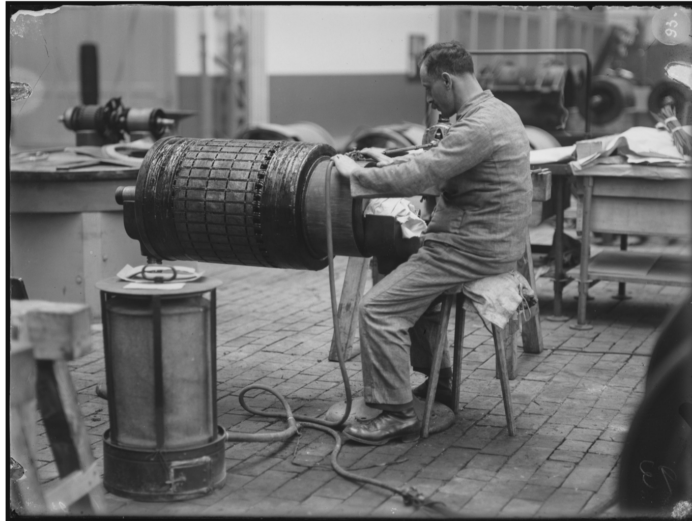
Worker assembling a locomotive transformer
