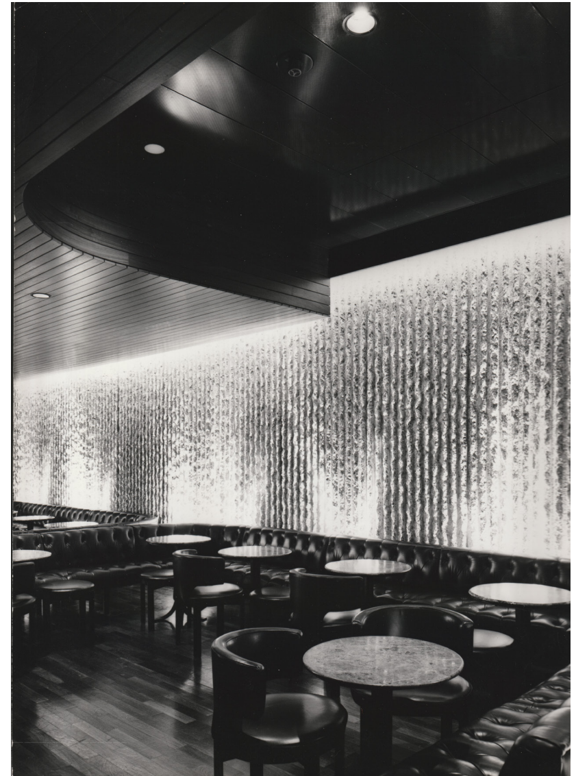
Traveller's Bar on ground floor, 1970's (Source: Archive Spögl)
