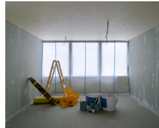
Guest room in renovation
