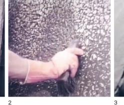
Shortly before the top cement skin is hardened, it is washed off with a weakly flowing waterjet.
