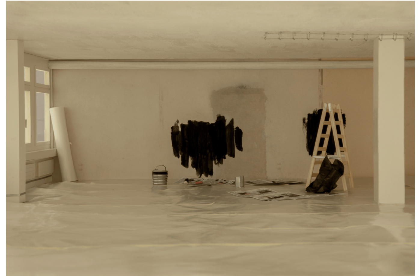
28.01.2021: starting the renovation process
