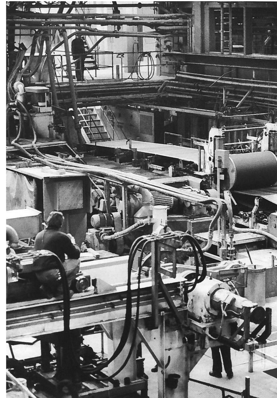
Eternit factory interior
