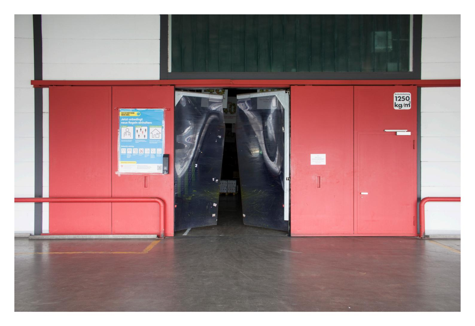
**D5.2** Separates: outside and internal street Function: transparent windbreak Time: 2 sec Material: plastic, galvanized steel Mechanism: human power Open: the whole day (00:00 - 24:00)
