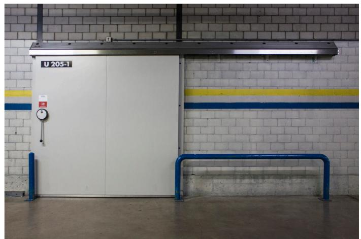
**D3** Separates: corridor and banana ripening Function: protection to ripen bananas Time: 1 min Material: plastic, steel, painted steel Mechnaism: motorized, lockable Open: through out the day (banana ripening takes up to 7 days)
