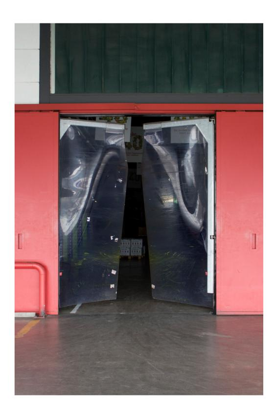
**D6** Separates: outside and rented storage Function: lock storage space Time: 25 sec Material: painted steel, profilit glass, plastic Mechnaism: motorized, lockable Open: 24:00 - 08:00; during the day when goods arrive
